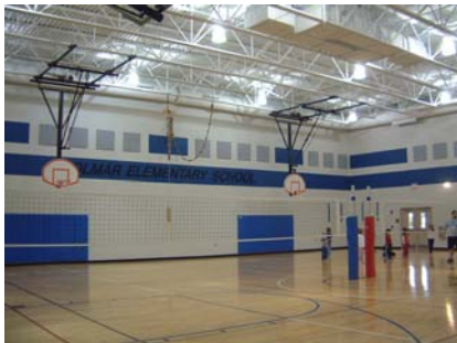
Absorption panels in an elementary school gymnasium
