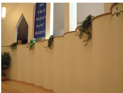
Diffused wall in a choir area at the front of a church
